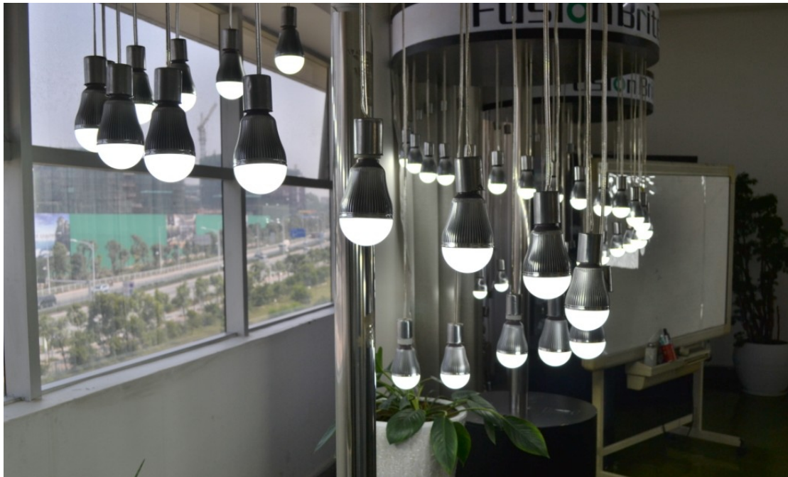
LED Ceiling Light Project in China
