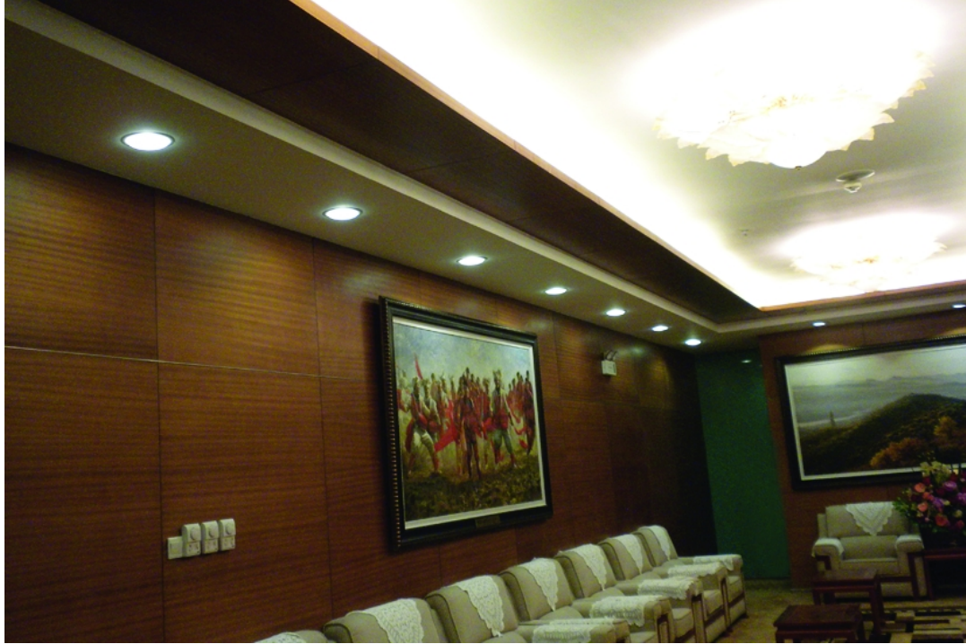
LED Down Light Project in China
