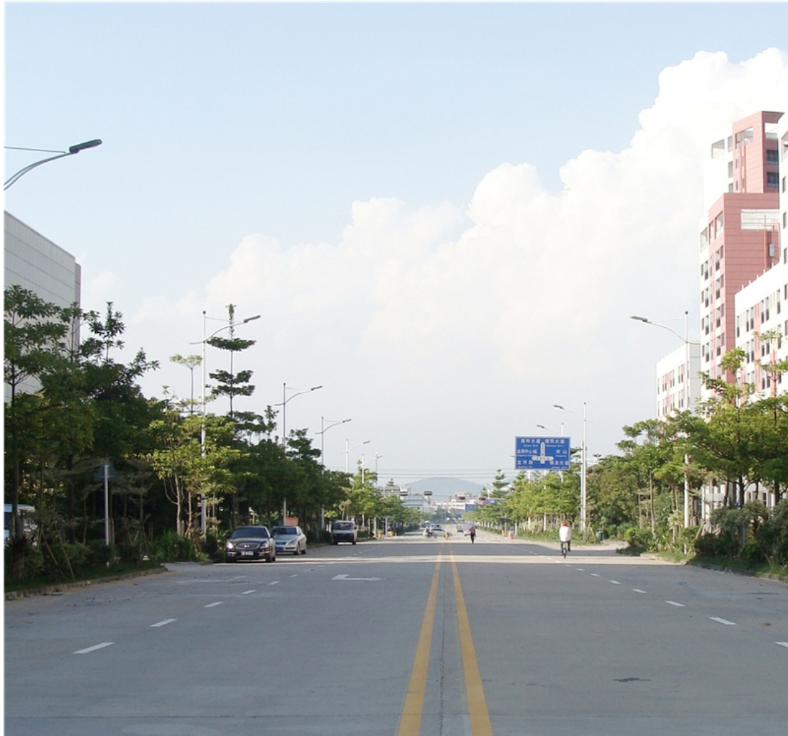
LED Street Light Project
