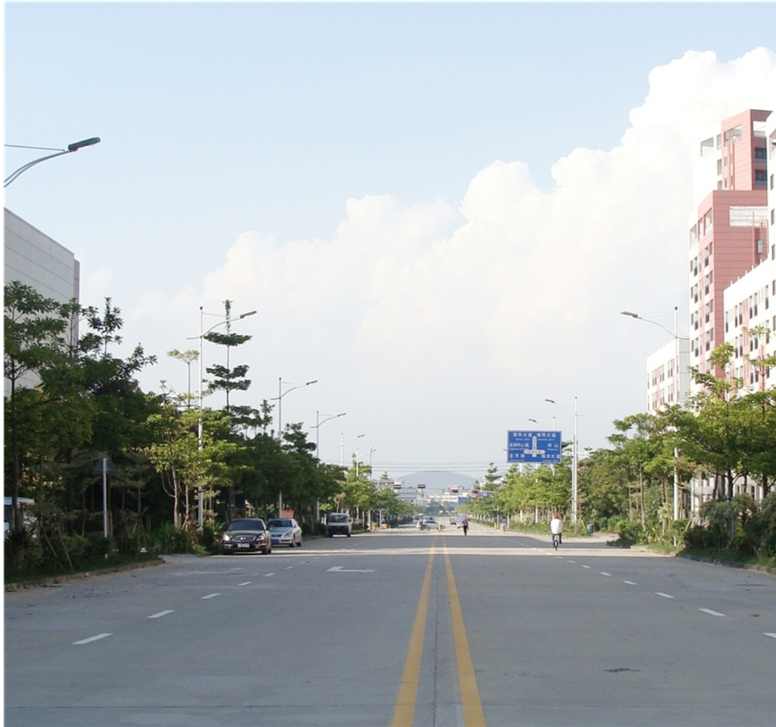
LED Street Light Project
